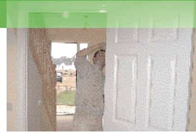
The finishing touches
